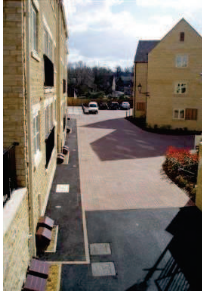
Permeable pavement, Stamford Robert Bray Associates
