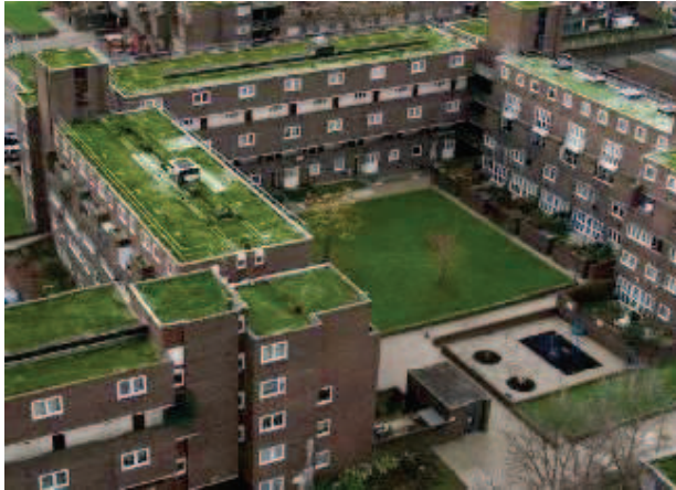
Green roof, London Lambeth Council
