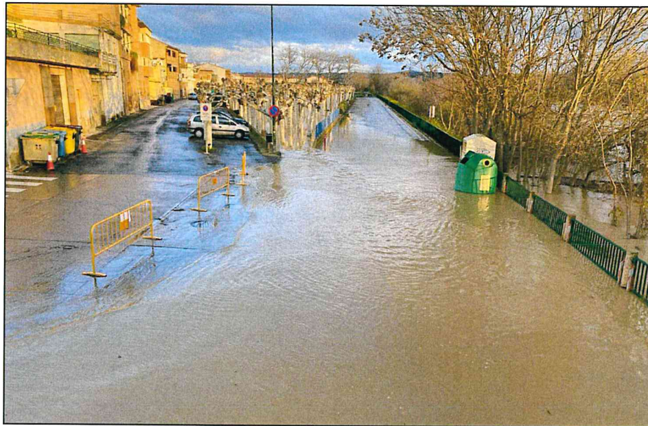
Paseo de la Mejana – low point in the right bank of the river, where flooding of the municipality starts.
