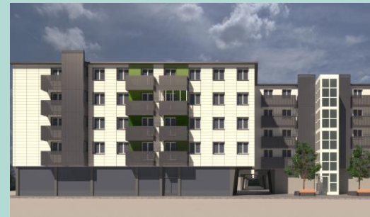
PIG n.28 (sept-2021) Plazas Rojas 16 buildings 128 dwellings Year of construction : 1971
