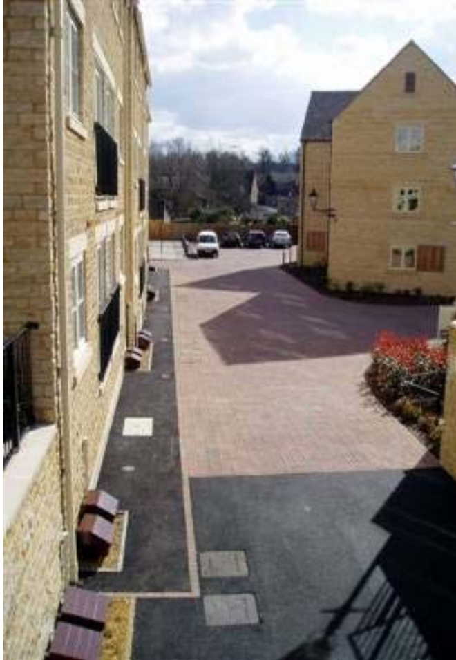
Permeable pavement, Stamford Robert Bray Associates
